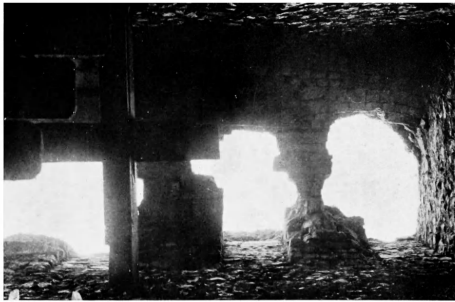
3. The above Arches from the floor
