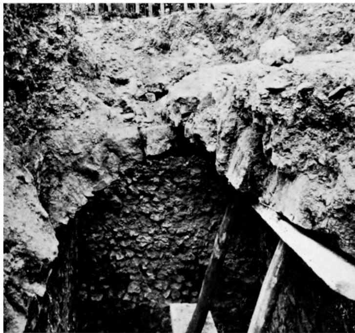
2. The front Arch and West wall LATRINE
