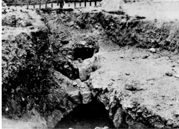
1. The two top Arches
